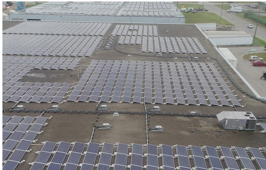
88 Todd, a 600kW DC Rooftop Solar Project.
